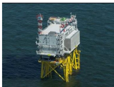
b) Fixed structure Jacket – installation
