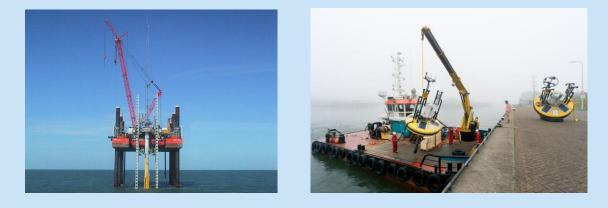
Source: Left: Installation of a met mast (Fugro Seacore); Right: Installation of a floating lidar device (RVO.nl).
